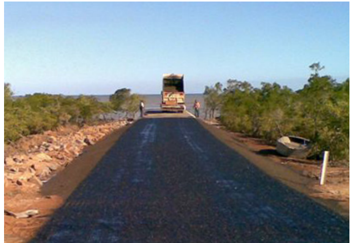
New Channel Point boat ramp under construction
